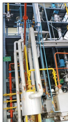
Falling Film Type Fraction Distillation Unit [250 Liters]
